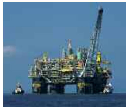
Petrobras P-51, the first semisubmersible production platform built entirely in Brazil: 48,000 tonnes and almost US$1 billion to produce 180,000 BOPD in 1,255 m of water, on stream January 2009
